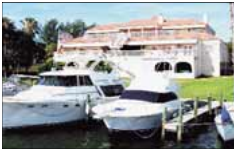
Safe Harbor's office in Longboat Key, Florida
